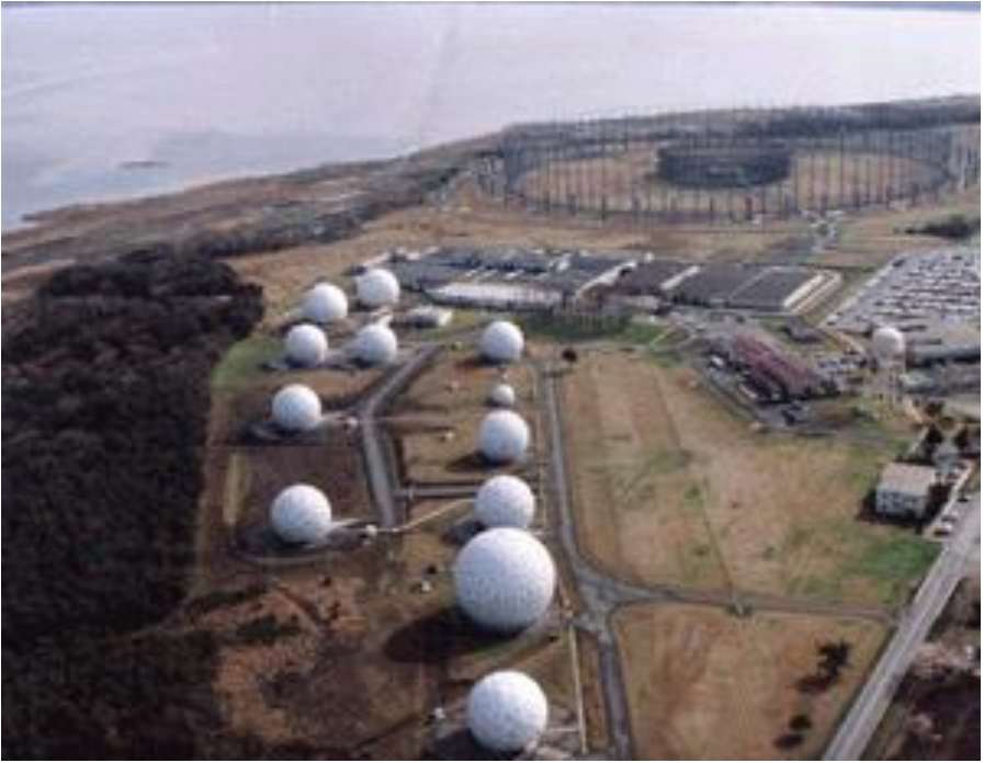
Misawa Air Base Security Operations Center, Towada, Japan
